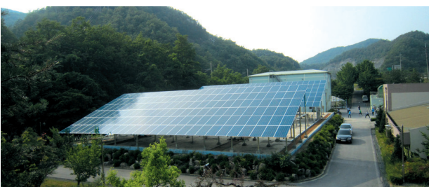
Danyang Wastewater Treatment Plant
